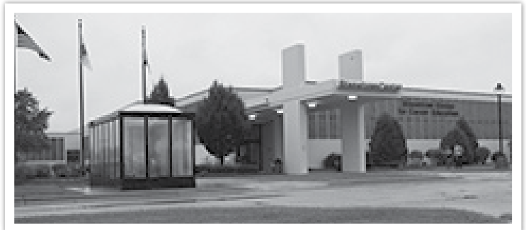
SAMUELSON ROAD CENTER (SAML) located at 4151 Samuelson Road, Rockford, IL 61109 just east of Rockford Jefferson High School
