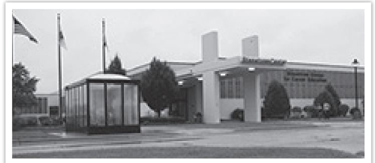
Stenstrom Center for Career Education (SCCE), formerly Samuelson Road Center (SAML) located at 4151 Samuelson Road, Rockford, IL 61109 just east of Rockford Jefferson High School
