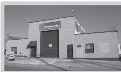
Cold Forming Training Center (CFTC) located at 424 Buckbee Street Rockford, IL 61104;
